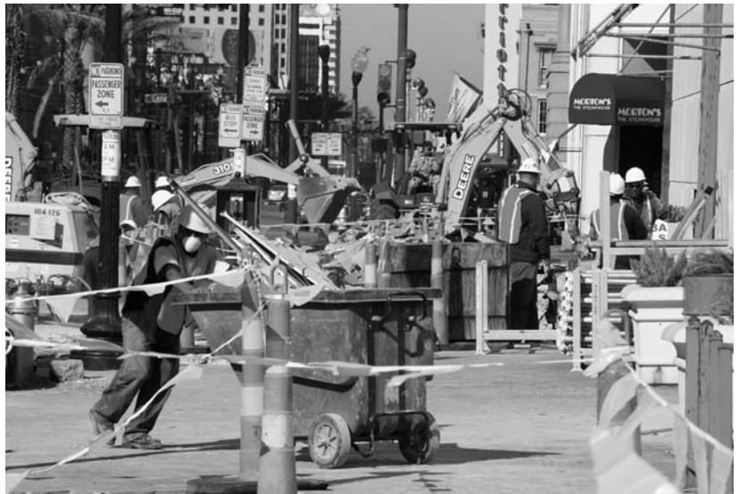
NEW ORLEANS, DECEMBER, 2005 Construction projects line New Orleans streets.
