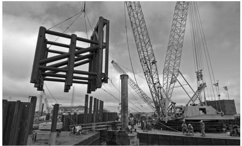
NEW ORLEANS, APRIL 2006 Construction underway at the 17th Street Canal.
